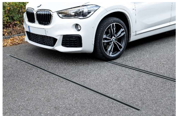
SL SPZ sensor installation
