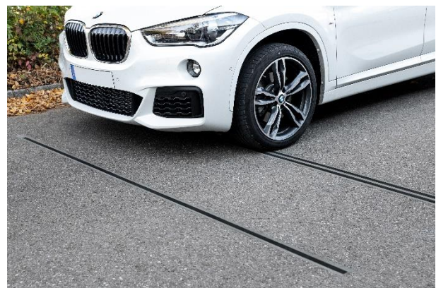
SL PUR sensor installation
